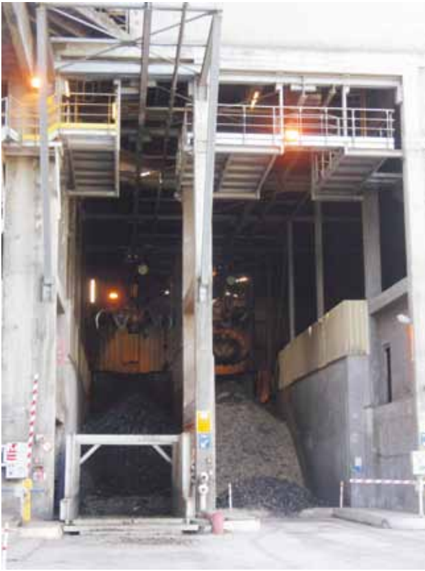
Figure 5. Unloading zone in the bunker and halls with automatic cranes. Manufacturer: ATS Group Water Materials Handling. (Source: MVW Lechtenberg).
